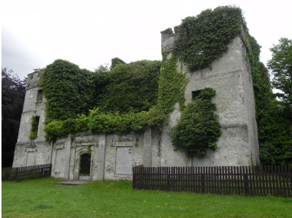
Fig. 19. Ivy, while of benefit to wildlife, can quickly come to dominate old walls, displacing smaller species and potentially causing structural damage. Photo: Donadea, Daniel Kelly.
